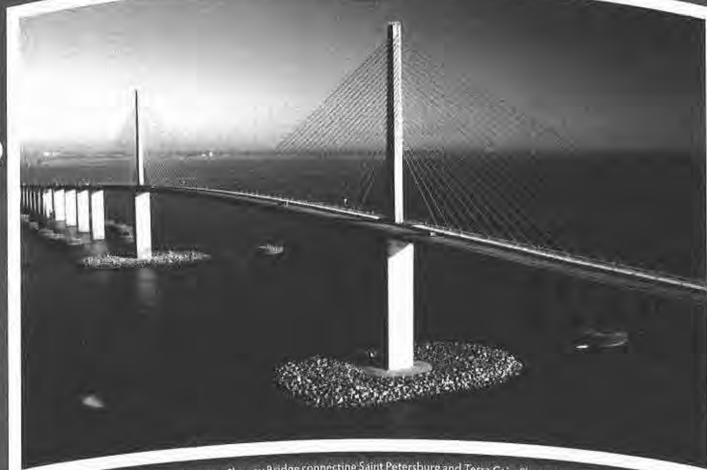
Sunshine Skyway Bridge connecting Saint Petersburg and Terra Ceia, Florida
