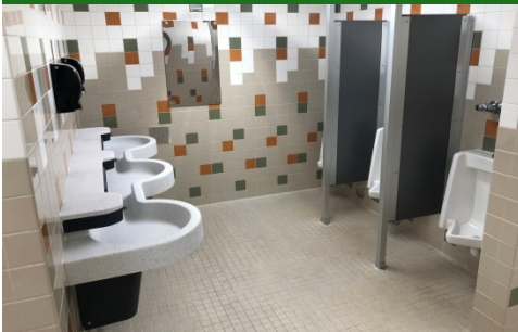
Building 14 In progress
