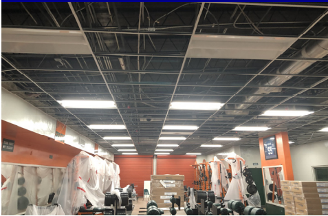
Building 2 In progress
