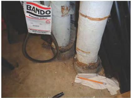
Photo 5: FISH 221A, Felt paper at bottom of pipes
