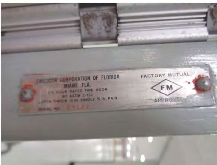
Photo 8: Typical fire door label
