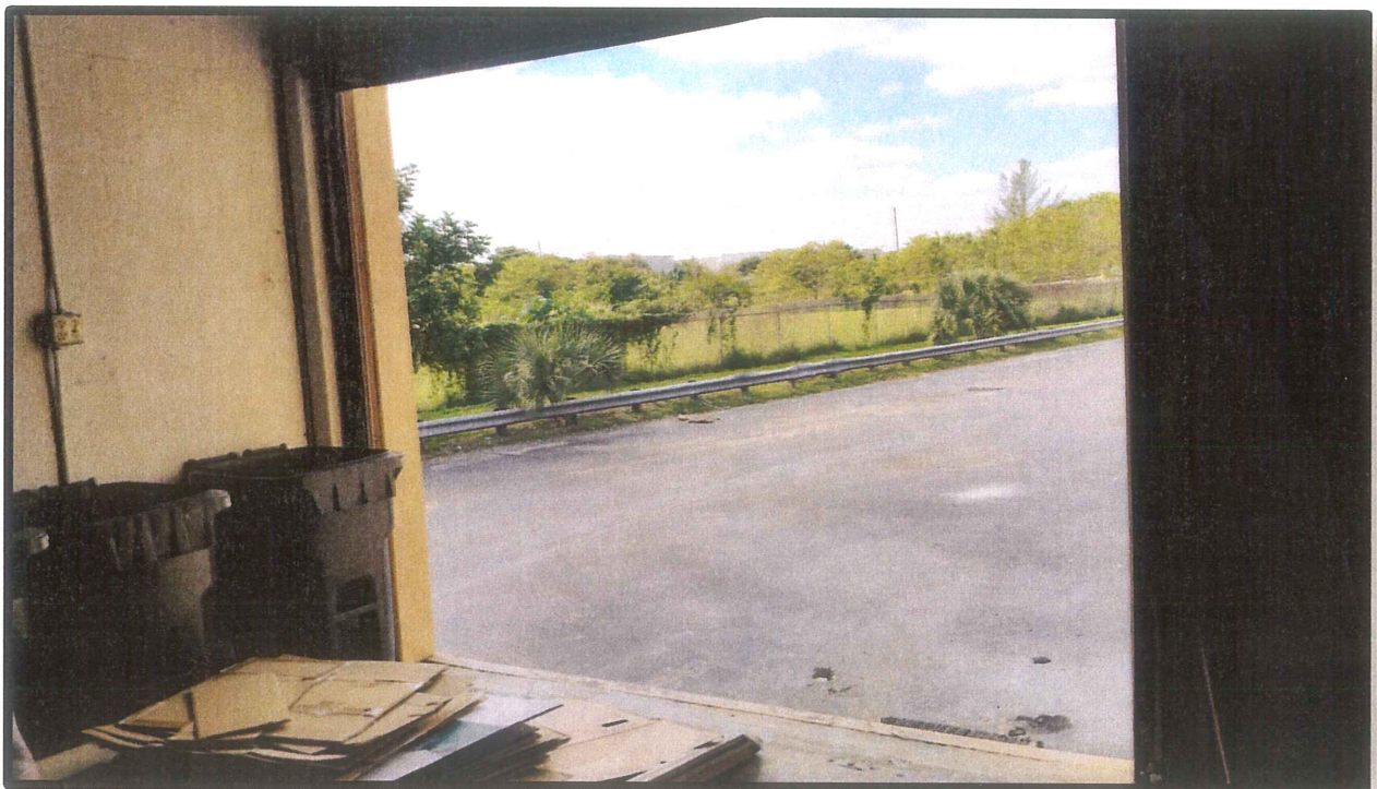
BEF PICTURE #2 - LOADING DOCK
