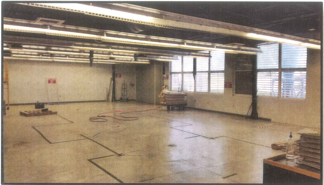
SHERIDAN PICTURE #3 - WOODSHOP CLASSROOM AREA HAS APPROX. 3,000 SF LOADING AREA
