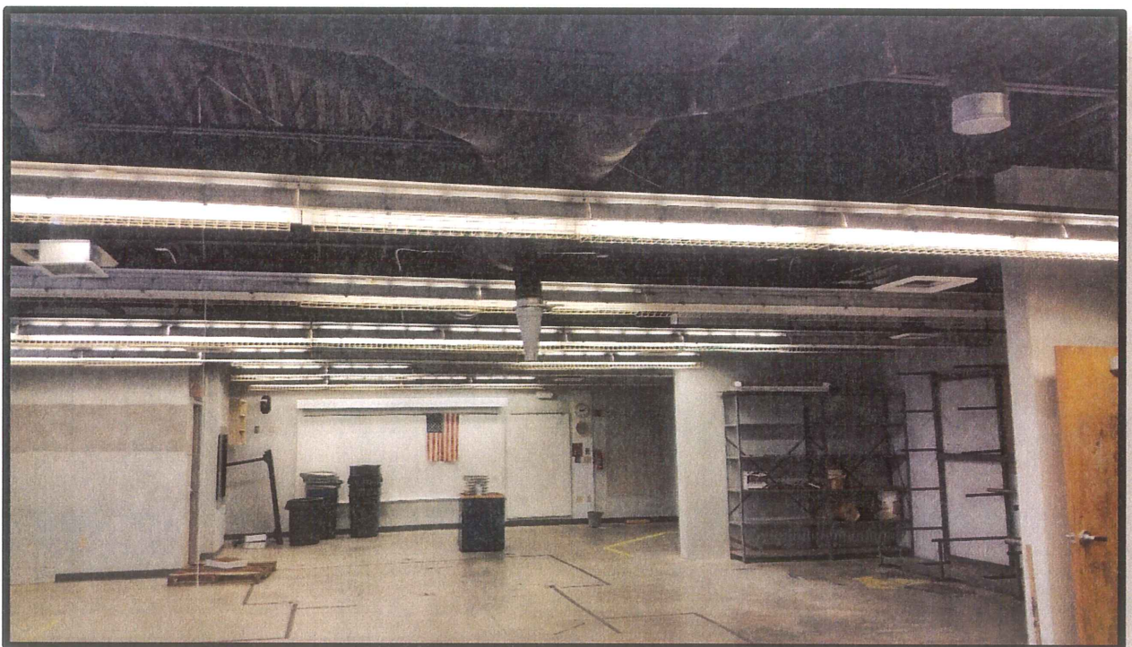
SHERIDAN PICTURE #4 - WOODSHOP CLASSROOM AREA HAS 12' FT. CEILING HEIGHT
